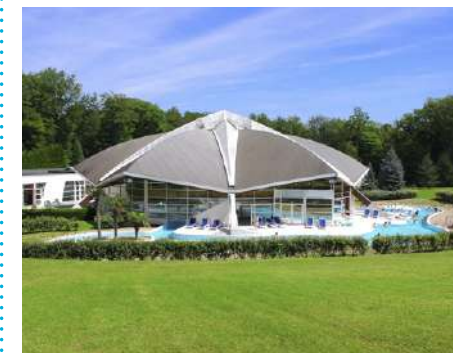
© POLE THERMAL AMNEVILLE
